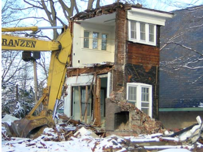
Demolition of 608 West Green Street, Urbana
